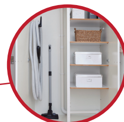
Pipe installation in cabinet
